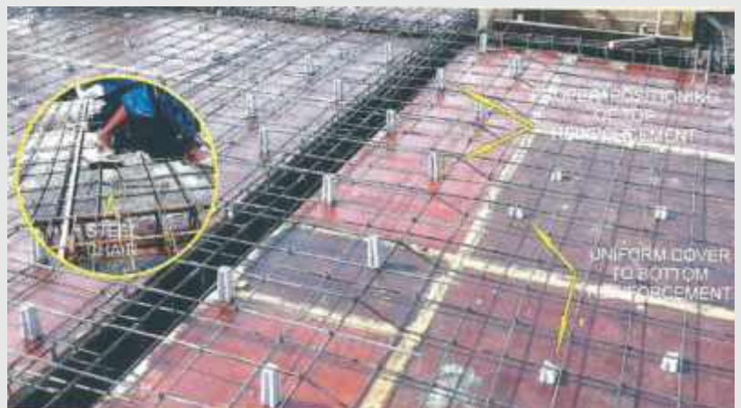
Spacers are most effective to position the reinforcement
